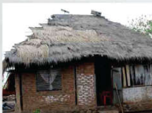
Solar Home System
