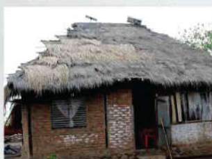
Solar Home System
