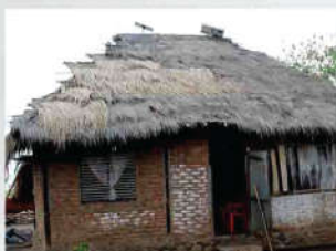
Solar Home System
